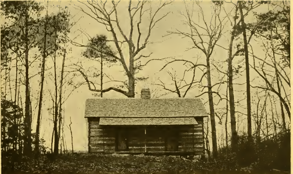
REPLICA OF THE BOONE HOME ON THE YADKIN RIVER IN NORTH CAROLINA Erected by the Daniel Boone Memorial Association.
